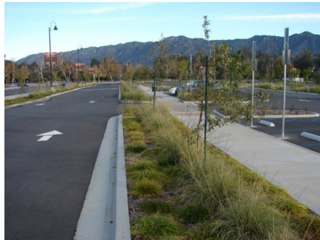
Figure 3.10 LA Zoo Parking Lot Stormwater Infiltration
