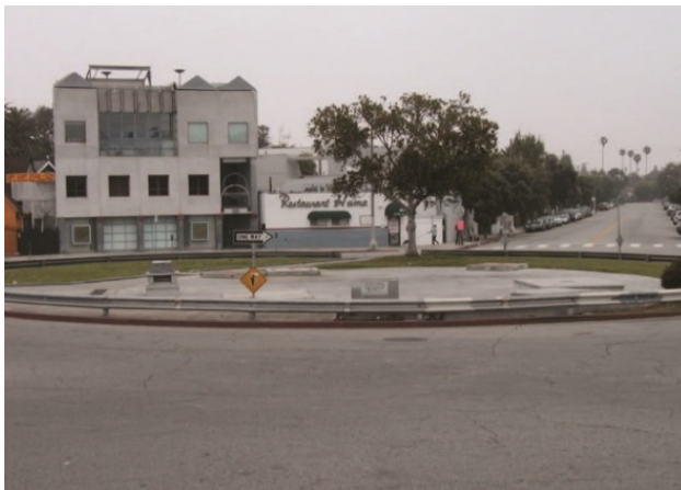
Venice Low Flow Diversion Pump Station
