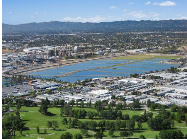
The Groundwater Replenishment Project will recharge up to 30,000 acre-feet of purified recycled water per year into the San Fernando groundwater basin at the Hansen Spreading Grounds (shown) and Pacoima Spreading Grounds for percolation.
