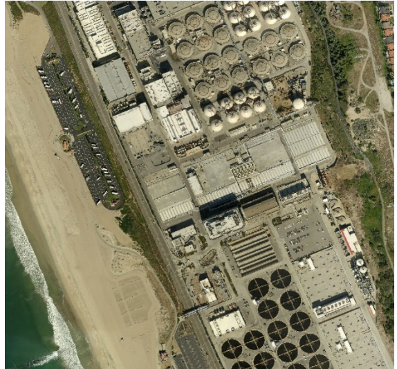
The City is assessing a wide variety of options to maximize recycling through regional collaboration and partnerships at Hyperion, the City's largest Water Reclamation Plant.
