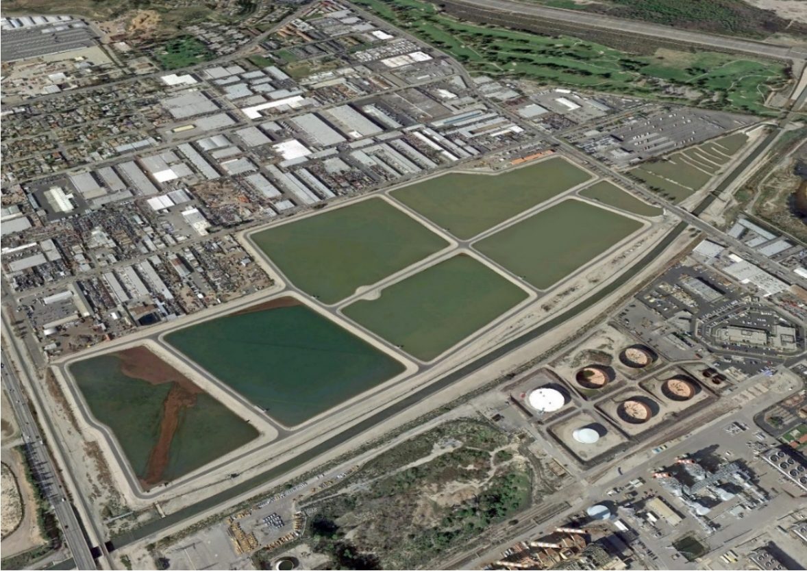
Figure 3.9 Hansen Spreading Grounds
